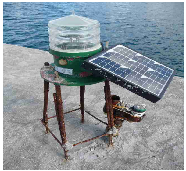
There is a beacon light furthest out that is powered by solar cells.
