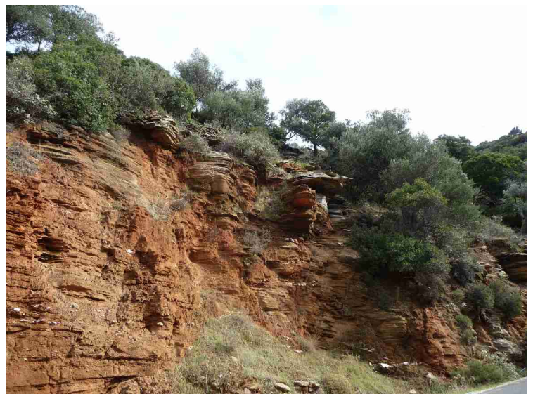
The roads have to be cut into the terrain.
