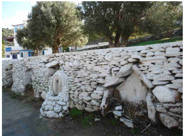
Wall with water tap
