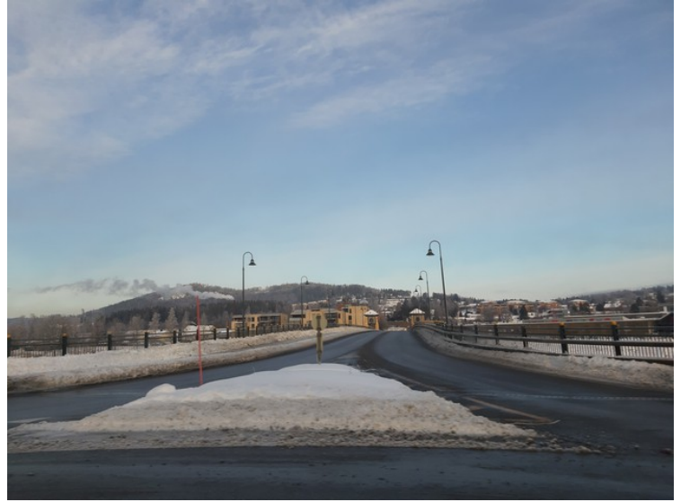
Here we have come to Gjemselund bridge in Kongsvinger.
