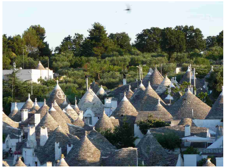
Many roofs on trulli houses
