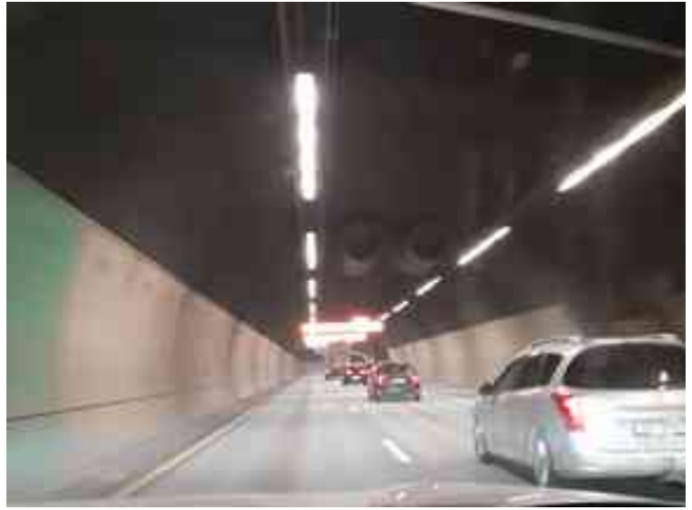
In the tunnel.
